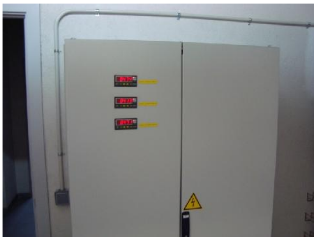
Monitoring, control and protection cabinet
