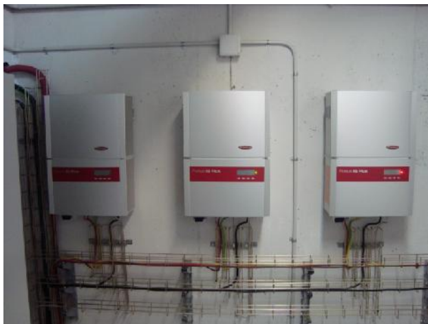
3 x 3,5 kW Single phase inverters
